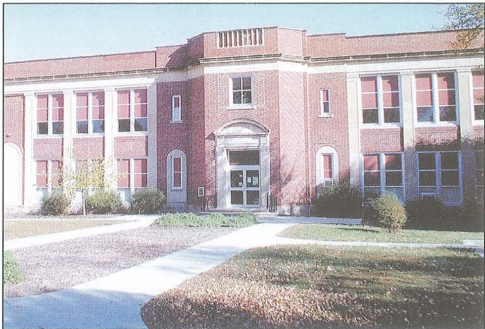
Encompass Architects is renovating Sheridan Elementary School.
