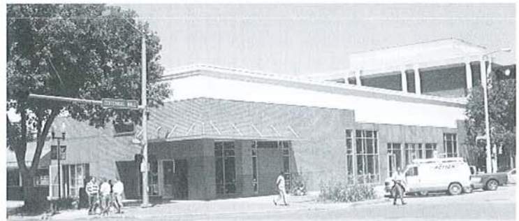
Below: After extensive renovation, the Rialto Building at 15 & O Streets houses four new retail bays, one of which will house Taco Bueno.
