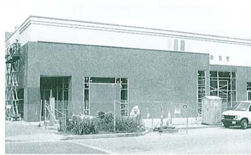
Renovation continues on The Rialto at 15th and O Streets
